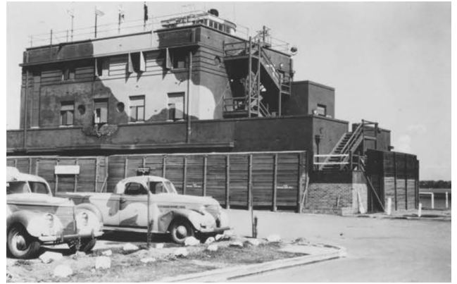
Note the camouflage and splinter proof walls on the Terminal building in Aug 1943.
