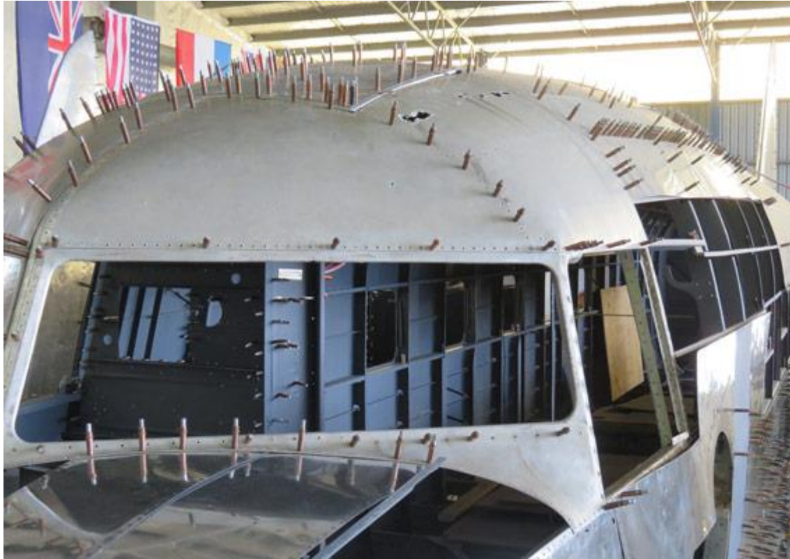
Skin pins around the cockpit of the DC2 temporarily replace rivets.
