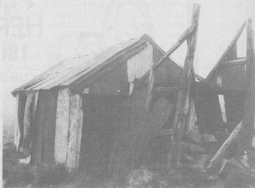
Rumpffs' Spring Hill hut, iron-sheathed and part derelict.
