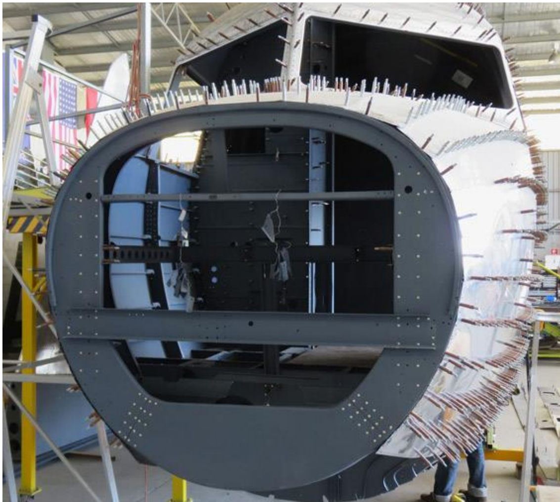
The nose frame was the last fuselage support to be riveted in place.
