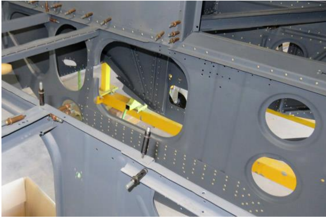
The last floor frame has been riveted into position
