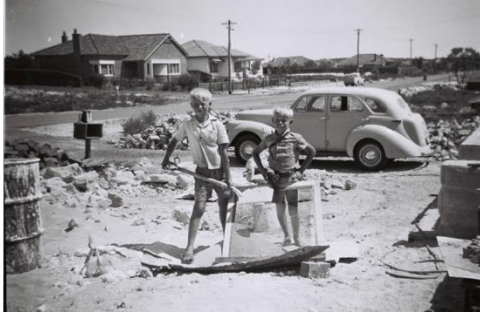
Cleaning bricks. Mixing cement to lay bricks
